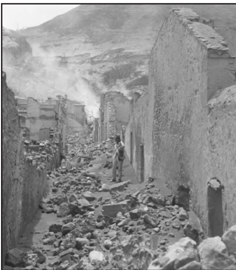
Rubble covers a side street in northern Saint-Pierre in 1902.
