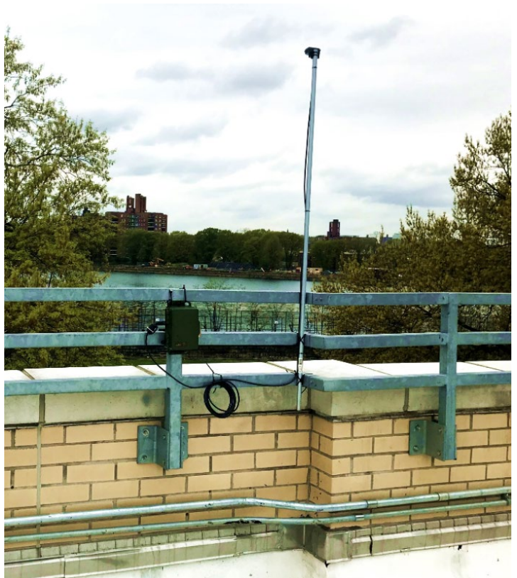
Figure 5. A typical set up for the SM4 Bat recorder and microphone—here, on a high school in the Bronx, NY. The further the microphone is away from other structures, the better. Ideally, microphones should be set at least 3 meters above the ground or (seen here) above the roof to minimize clutter in recordings. Clutter is the reflection of pulses off nearby hard surfaces that can obfuscate, or "clutter" recordings—making them more difficult to interpret.
